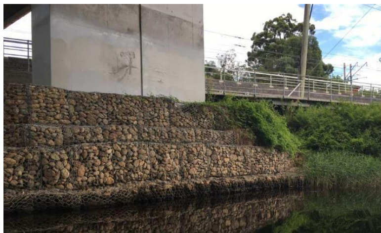
RHDHV (2017) also reported scour protection works associated with the abutments of the M5 bridge over the Georges River (Figure 15).
